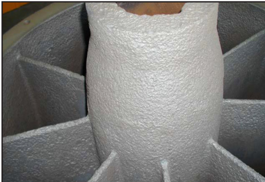
Pump diffuser after removal of old coal tar epoxy coating
